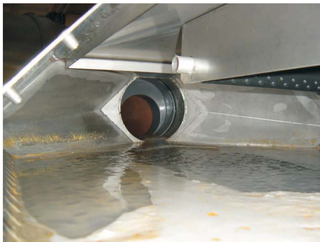
Fercher Wastewater Heat Exchangers Type AWT-928, inside view
