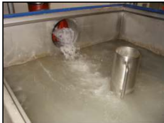
Photo: Wastewater distribution basin inside the FERNETT Wastewater Heat Exchanger
