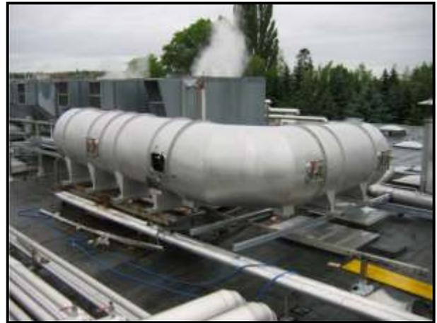
Photo: Fercher Energy Spray Tunnel Type EST-D-1800
