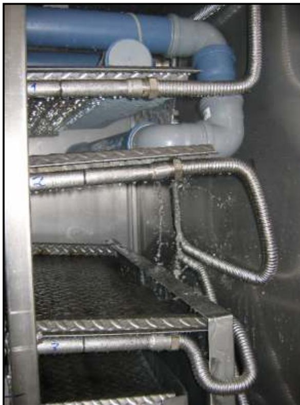
Photo: FERCHER Wastewater Heat Exchanger Type FB-8/S during operation
